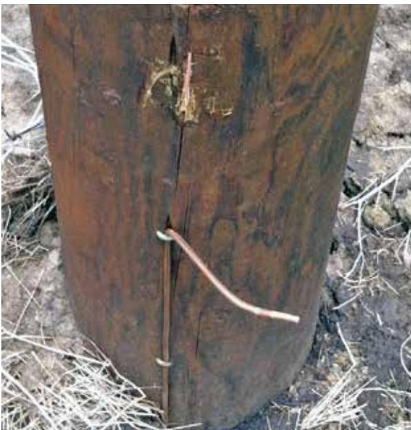
**A close-up view of a cut ground wire.**
